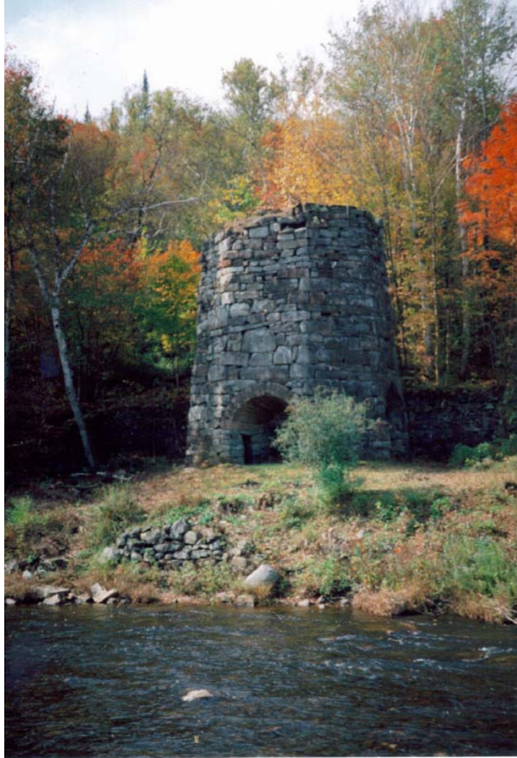
The only 'blast' furnace still standing in New Hampshire is located in Franconia on the banks of the Gale River. This iron works used to produce pig iron using iron ore and charcoal in the 1800s. (Photo courtesy of the Franconia Heritage Museum)
